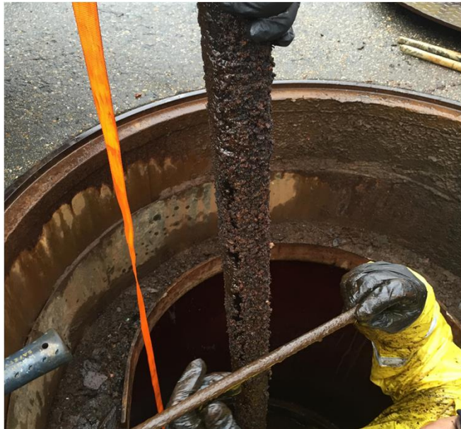
Corrosion on Submersible Turbine Pump
